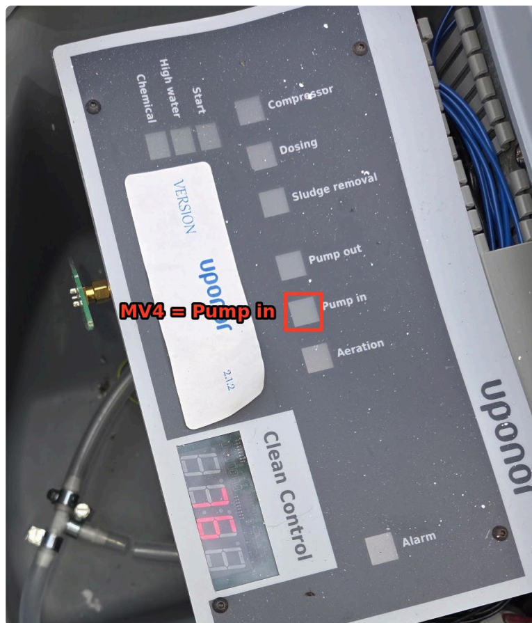
The Pump in light on the lid is on during the first step of the test cycle
